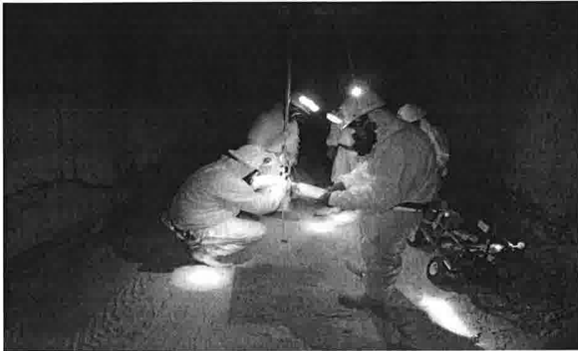
Figure 1: Geomechanical engineers in PPE, taking convergence measurements in a contaminated drift
