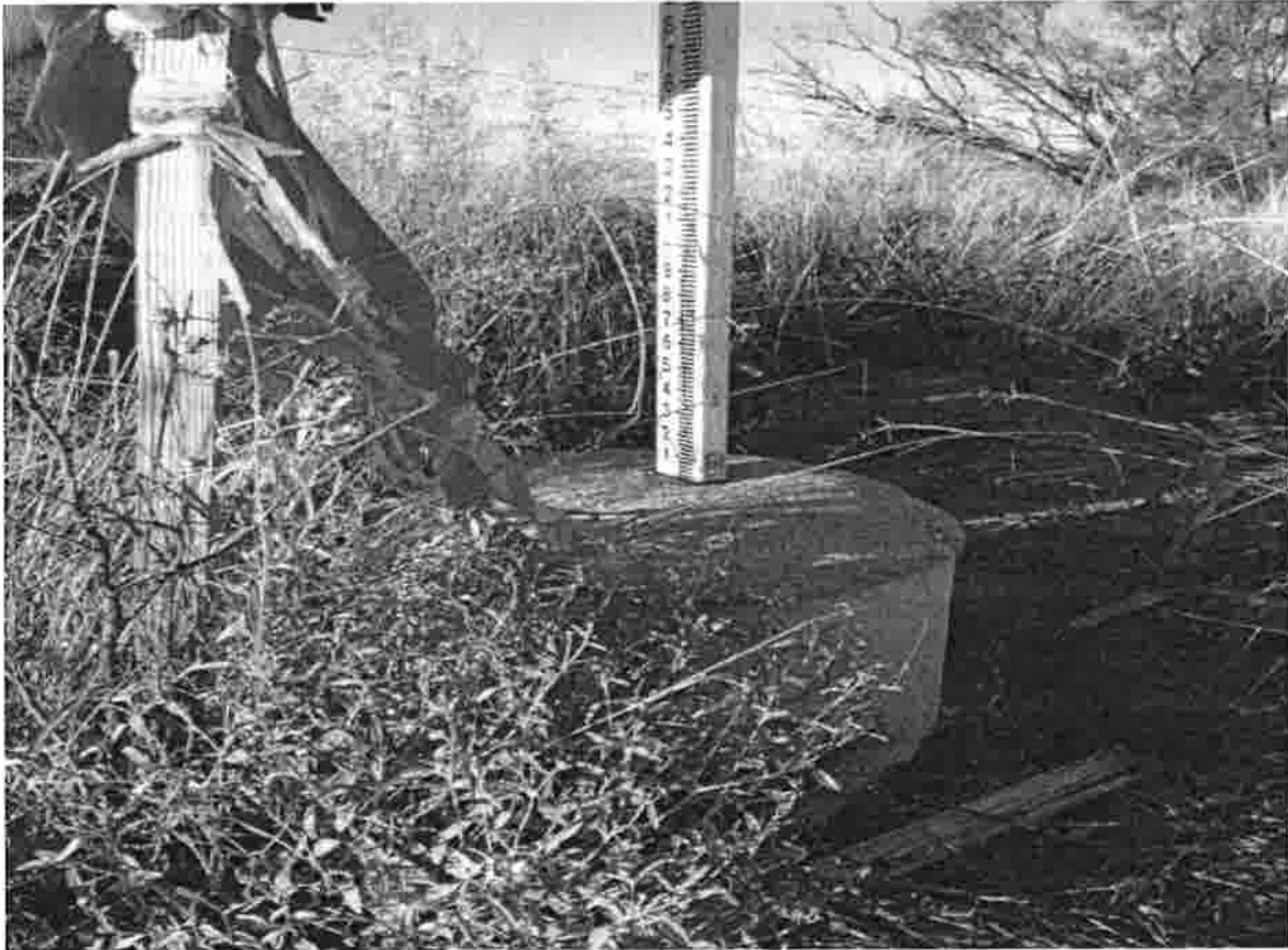
Figure 3. Surveying Rod on Monument S-24, taken during 2013 inspection.
